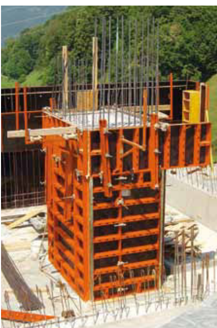
Neubau Skistation, CH-Oberterzen; Fa. Toneatti AG, CH-Bilten
